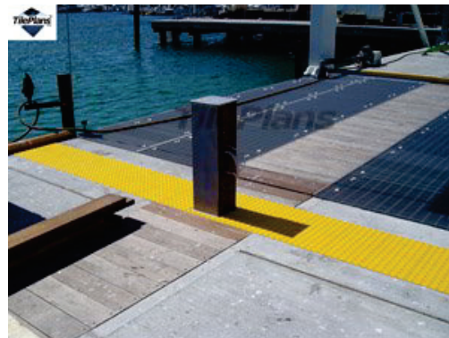
Tactile Paving installed in Yellow
